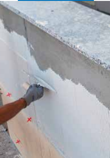
Laying on an external façade: application of adhesive on the substrate
