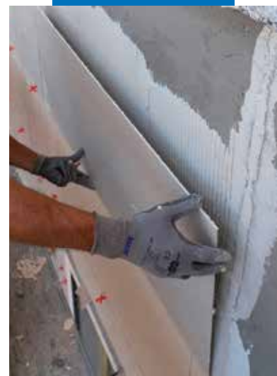
Applying a thin porcelain tile on an external façade
