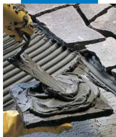
Installation of external hewn back stones with or without buttering, depending on thickness
