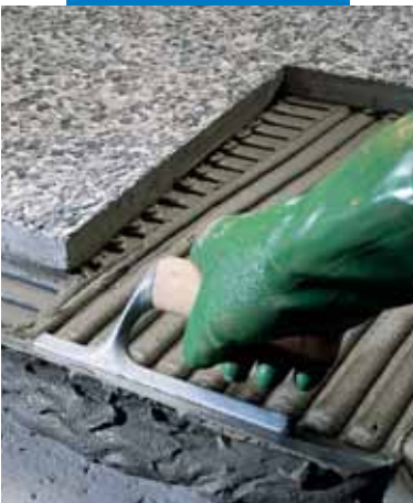
External installation of relief terrazzo "graniglie" tiles
