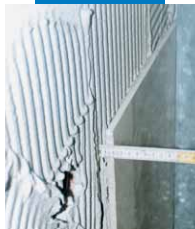
Thickly applied porcelain tiles on a wall
