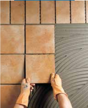
External installation of klinker tiles
