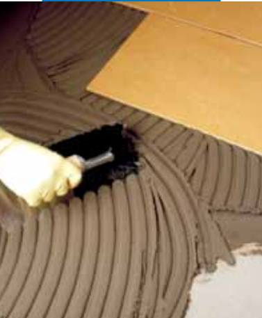
Spreading Elastorapid on a cementitious screed with a notched trowel
