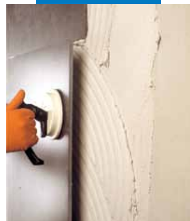
Laying large-sized porcelain tiles on a concrete façade with Elastorapid
