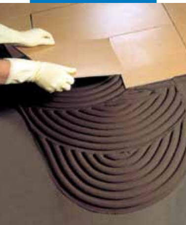
Laying porcelain tiles on a screed waterproofed with Mapelastic
