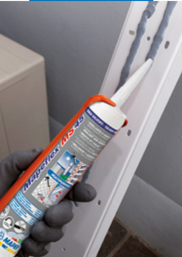
Bonding plastic profiles on a surface outside
