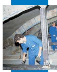
Pouring Mapegrout Hi-Flow into metal formwork
