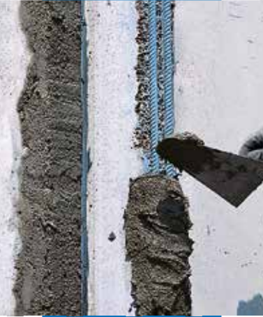
Application with trowel
