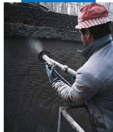
Bertini hydroelectric canal - Robbiate (Como) - Italy: spray application
