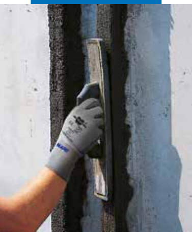
Finishing with a sponge float
