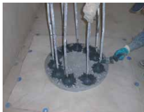
Fig. 2 - Application of Mapeproof Mastic around reinforcement rods in pile heads
