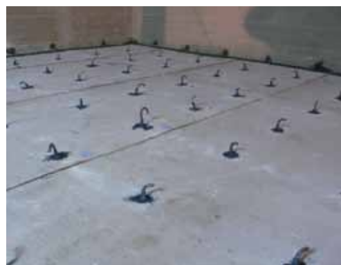
Fig. 4 - Grouting connection rods with Mapeproof Mastic
