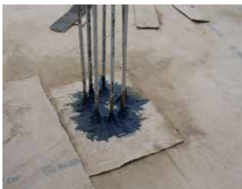
Fig. 3 - Sealing a piece of Mapeproof sheet around steel reinforcement rods with Mapeproof Mastic
