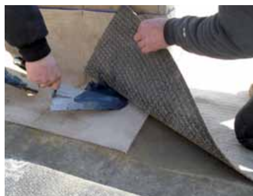
Fig. 6 - Sealing between Mapeproof bentonite sheets with Mapeproof Mastic
