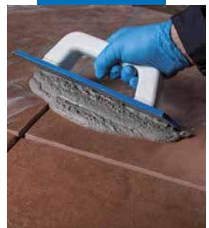
Grouting tiles with Ultracolor Plus
