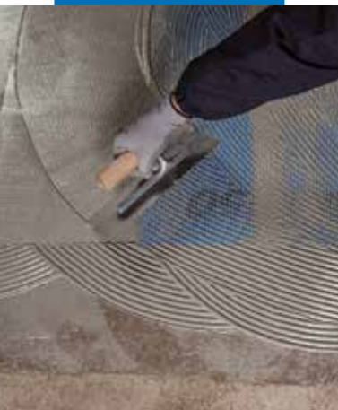
Placing Mapenet 150 on the first layer of Mapelastick Turbo while wet
