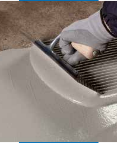
Application of the first layer of Mapelastick Turbo
