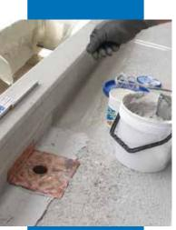
Laying a copper neckflange and drain spout
