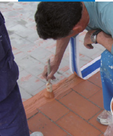
Waterproofing a distribution joint with Mapeband fixed in place with Aquaflex Roof
