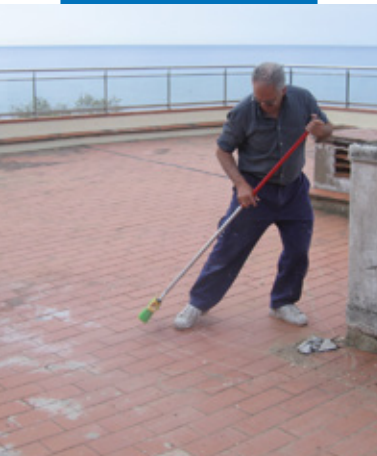
Cleaning a substrate before applying Aquaflex Roof
