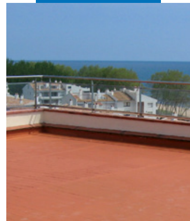
Paving slab waterproofed with Aquaflex Roof
